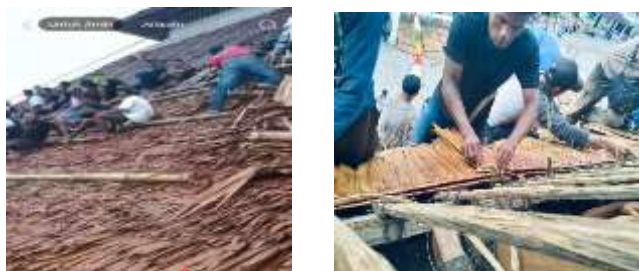
Figure 3. The Installation of The Mosque Roof Begins From The Bottom and Continues Upward.
